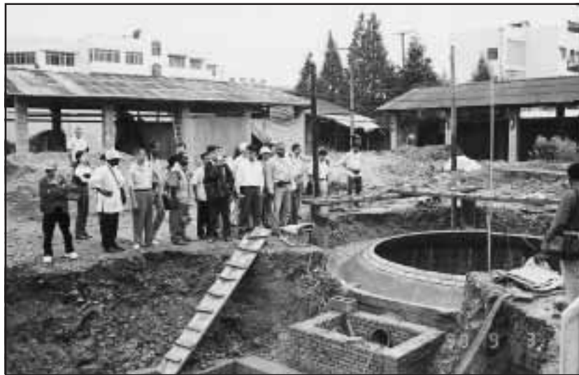
A Chinese Biogas Septic System with 120 m 3 under construction in Chongzhou City, Chengdu, Sichuan, China, September 1998. Photo by: Wu Libin, CBS.
