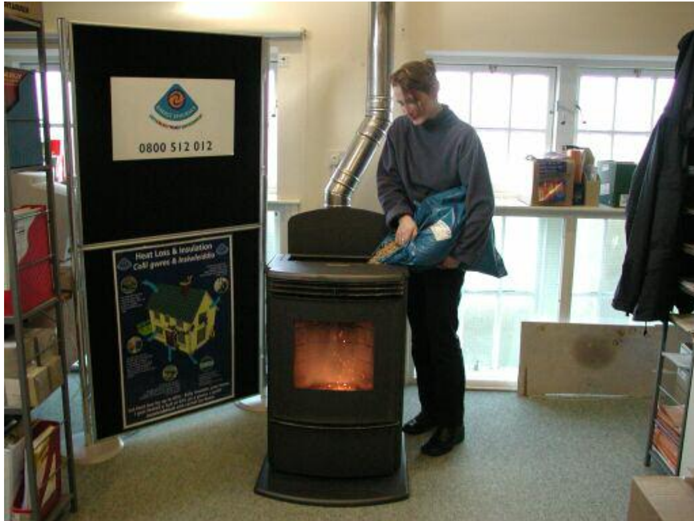
Wood pellet stove in our EEAC office (3kW to 11kW)
